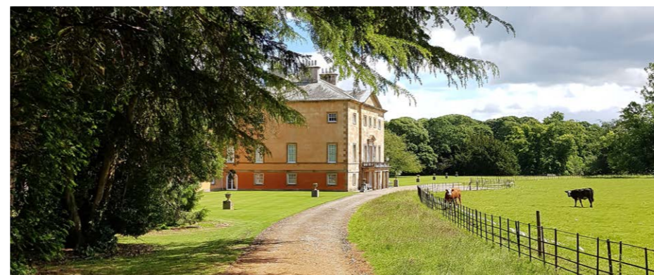
Plate 2: Grade I Listed Rokeby Park (house)
