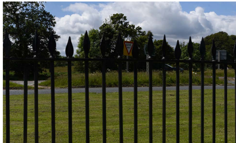
5 View from the Grade II listed piers and railings looking south west to the A66
