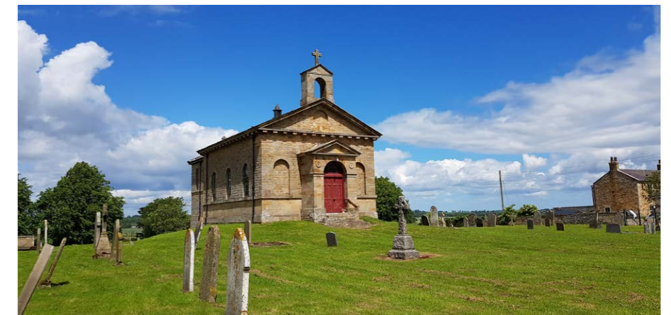
Plate 3: Grade II* Listed Church of St Mary
