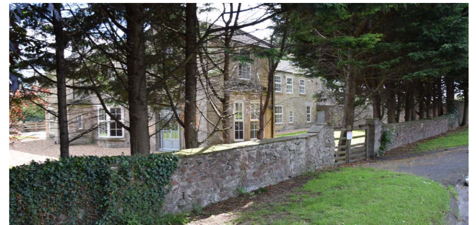
Plate 12: The Rectory, close to and below the west-bound carriageway
